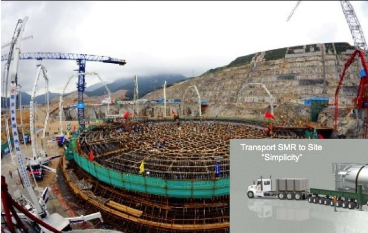
On-site Construction – “Complexity”
